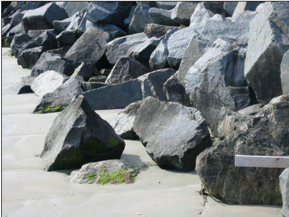
Figure 13. Photograph near north end of seawall, 11 February 2005. Individual stones have been displaced during storms.
