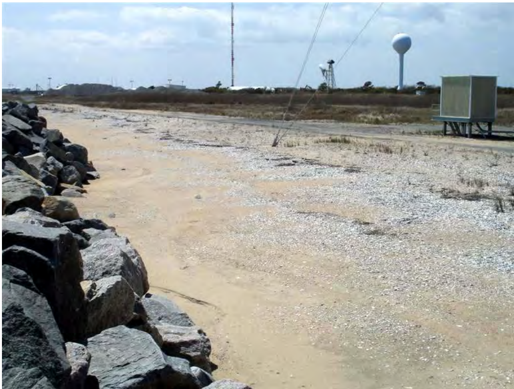
Figure 20. Back side of seawall south of U.S. Navy Aegis facility (Building V10/V20), 18 April 2006. Shell fragments and seaweed debris show approximate limit of wave uprush. View looking south.
