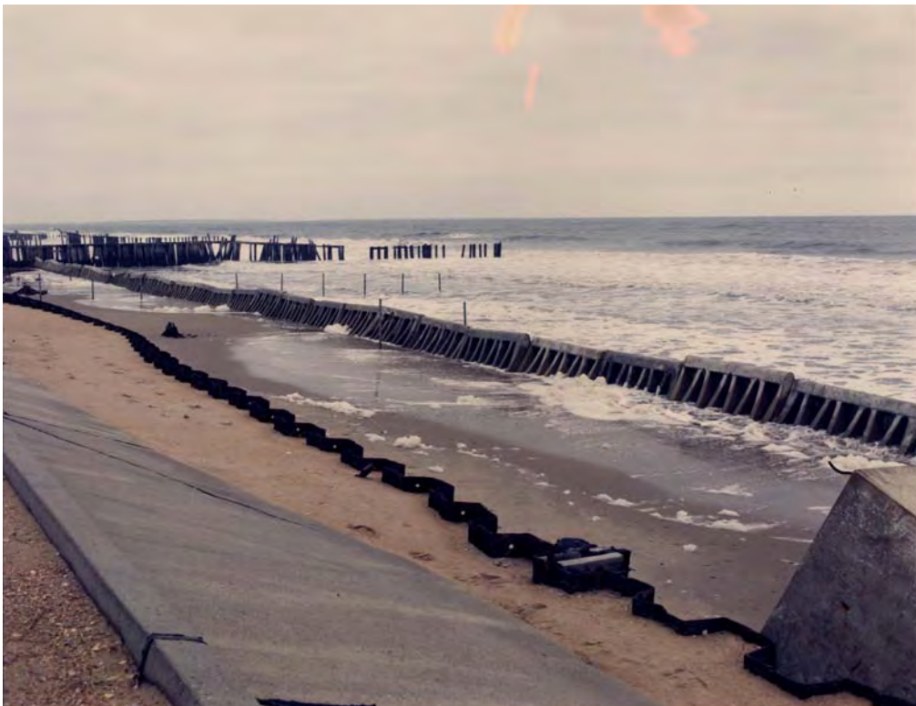
Figure 19. "Beach Beam" units partially sunken into seabed during an April 1988 storm.
