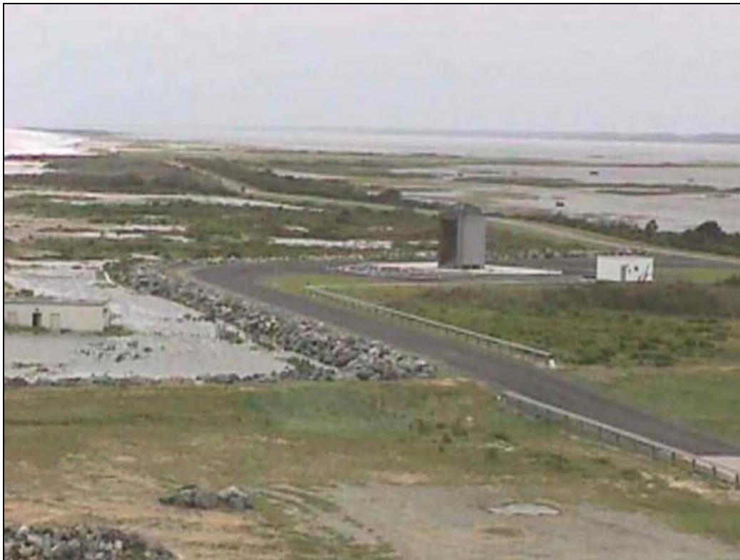
Figure 15. South end of Wallops Island during Hurricane Dennis (photograph taken approximately 1-4 September 1999. Standing water has reached the revetment in front of Pad 0B.
