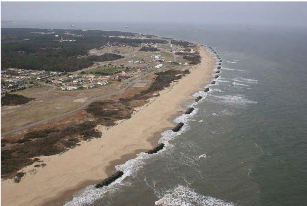
Figure 30. Breakwaters at Fort Story, VA, 31 March 2005. These were designed as headland breakwaters and built from land.
