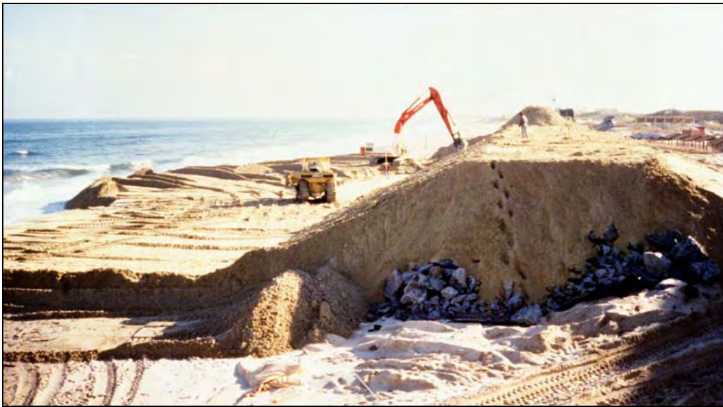
Figure 26. Construction of rock core dune at Dam Neck, VA (from Basco 2006)
