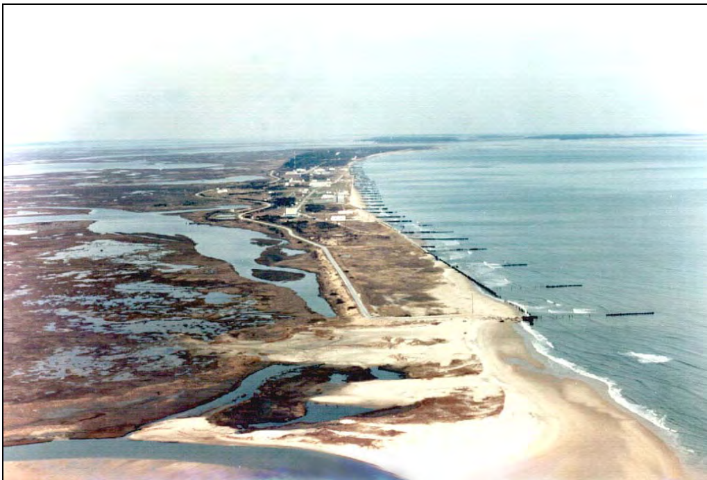
Figure 9. 1983 view looking north along Wallops Island showing poor condition of southern groins. NASA photograph 83-102-14, courtesy of Goddard Space Flight Center.
