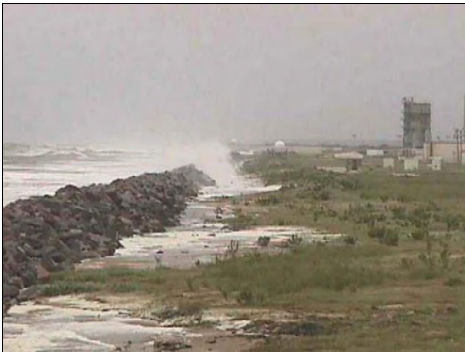
Figure 14. Waves from Hurricane Dennis overtopping the seawall (photograph taken approximately 1-4 September 1999).
