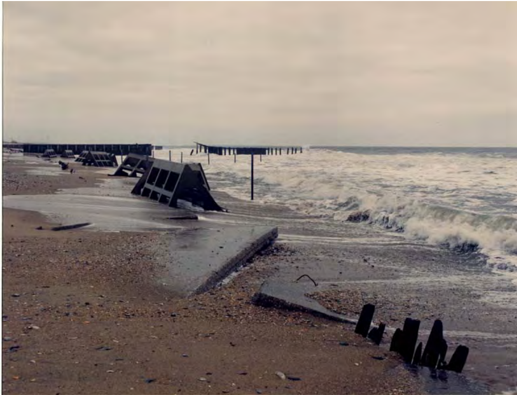
Figure 18. Experimental "Beach Prism" sand retention units moved out of alignment during an April 1988 storm (photograph courtesy of NASA).
