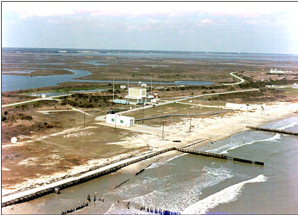
Figure 10. 1983 view taken in same area as Figure 7. Part of wood seawall has collapsed. NASA photograph 83-102-14, courtesy of Goddard Space Flight Center.
