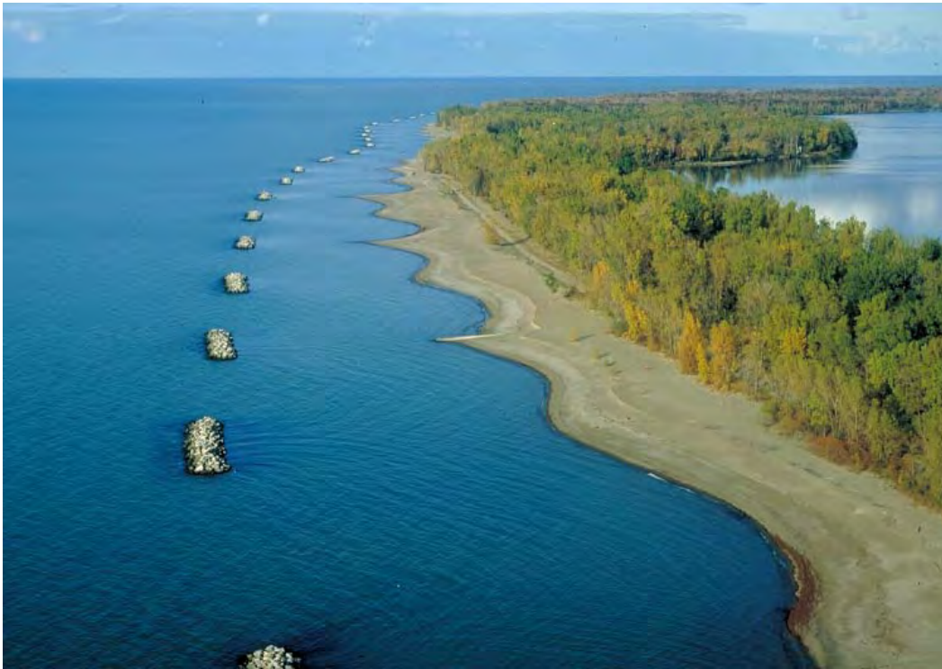
Figure 29. Detached breakwaters at Presque Isle, PA, in Lake Erie (from Mohr 1994). Since this photograph was taken in 1994, many of tombolos have grown out almost to breakwaters.
