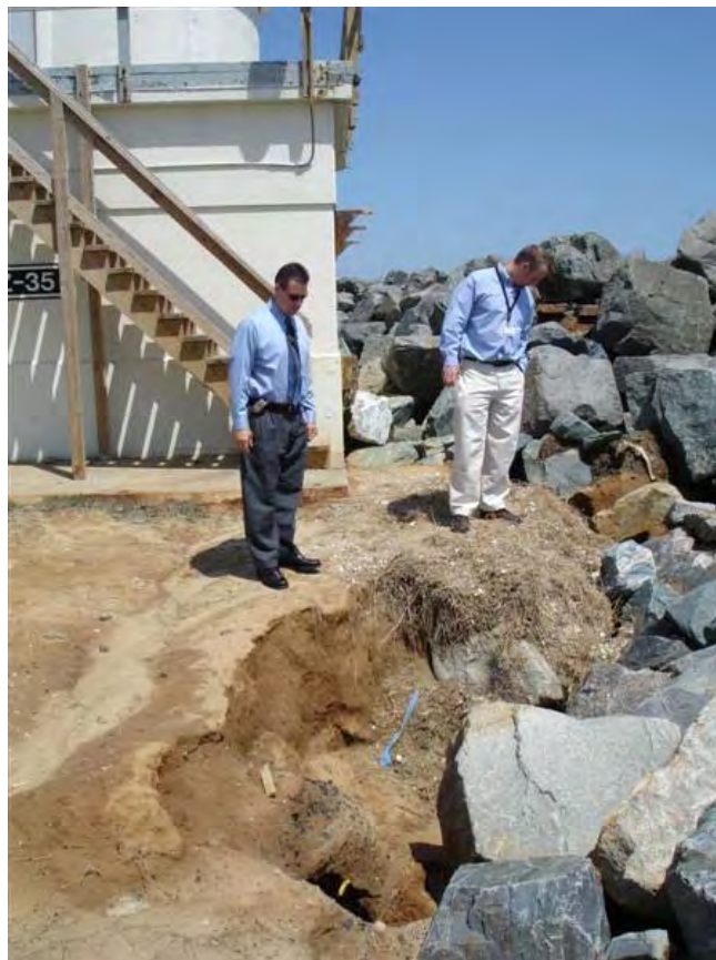
Figure 23. Sand loss at base of camera sta Z-35, 18 April 2006. To prevent foundation damage, NASA will install sheet pile and backfill, ocean is only 7 m to right beyond seawall.
