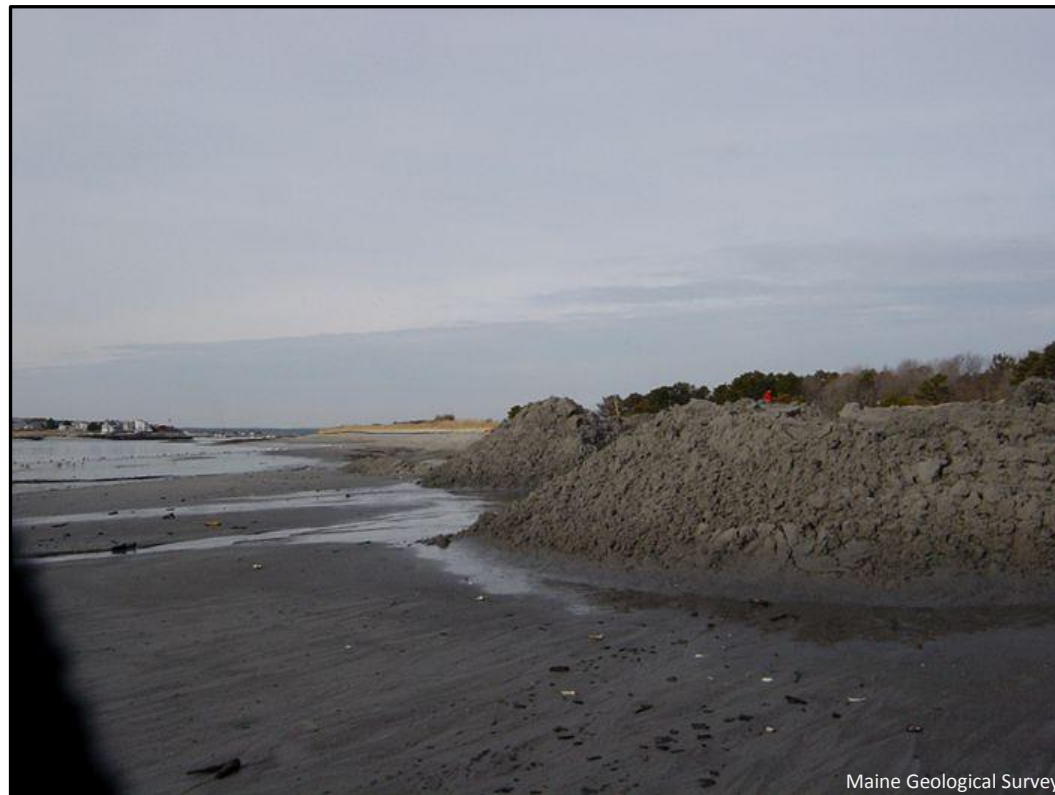
Figure 12. Photograph of mounds of dredged material on Western Beach prior to grading with equipment.
