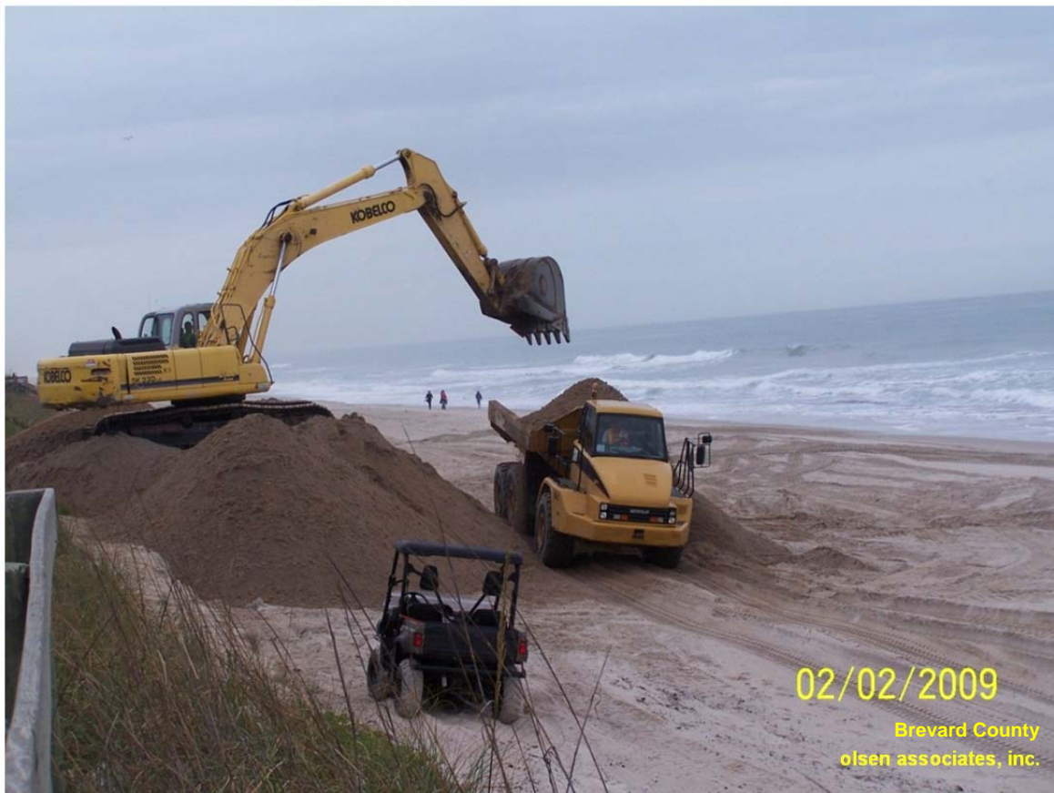
Figure 5.5b: Excavator moving material from a stockpile to an off-road dump truck.
