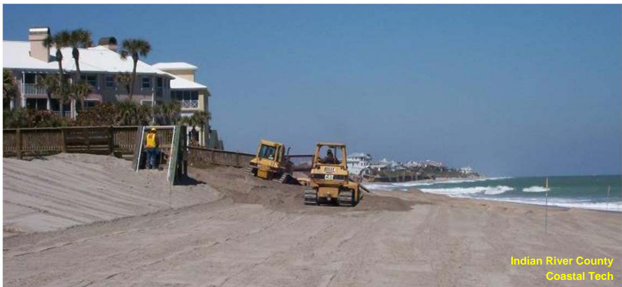
Figure 5.5d: Two dozers grooming fill sand to design specifications.
