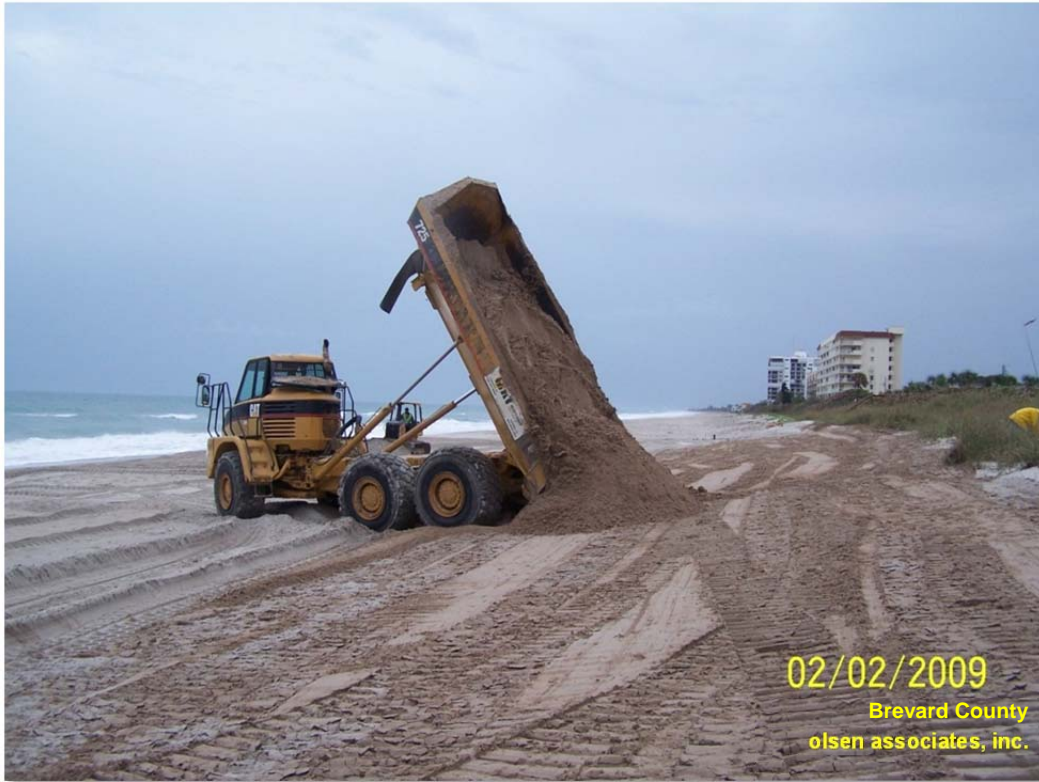
Figure 5.5c: Off-road truck dumping sand on the beach where it will then be spread and groomed by a dozer.
