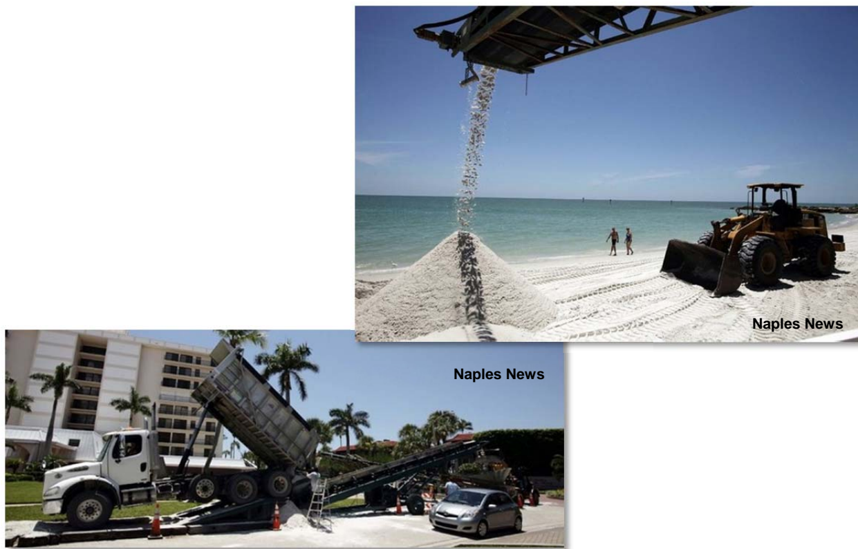
Figure 4.4: Transporting material to the beach via conveyer belt at a project in Collier County in 2010.
