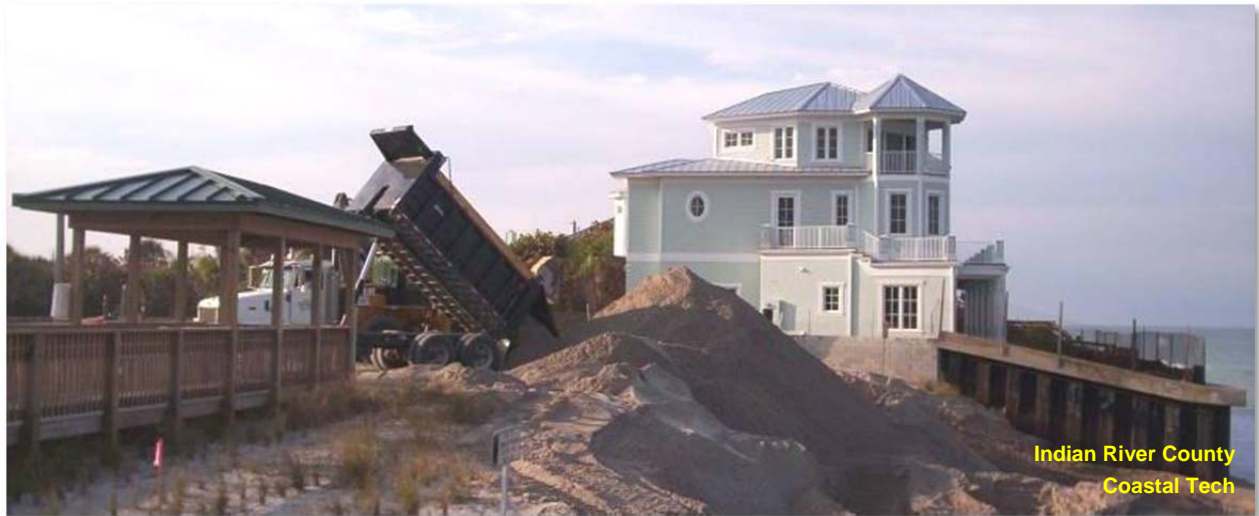
Figure 5.5a: Long-haul road truck dumping its sand load into a stockpile staging area.
