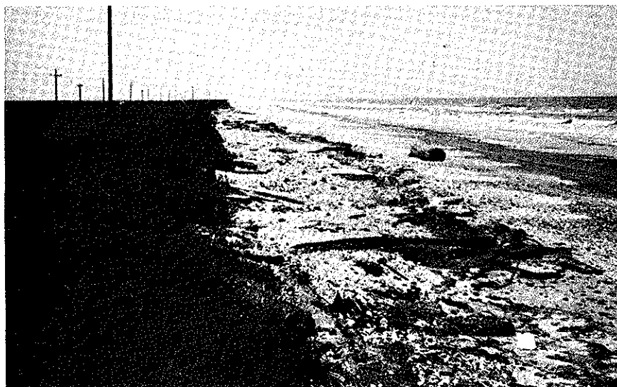
Plate 2. Remnants of a former roadbed of Highway 87. Trend of present highway is indicated by telephone poles in left background.
