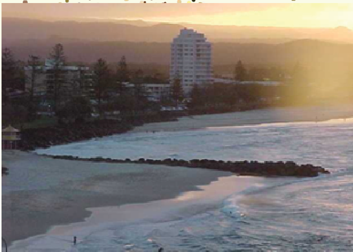
Figure 2. Groyne at Kirra Beach during the 1990s: sand builds up on the southern side of the groyne as longshore drift is interrupted. Note the erosion on the northern side of the groyne where the boulder wall is exposed.
