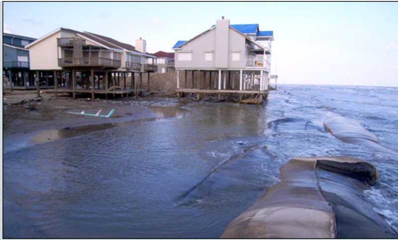
2008 Hurricane Ike slams into the Texas Coast, causing large-scale erosion to coastal communities. This image shows houses and erosional barriers (geotubes) exposed to the surf after wind and waves swept away beach sand.
