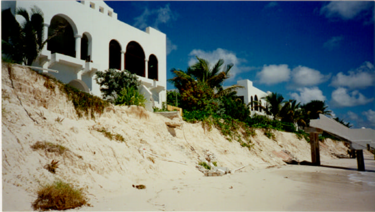
Photograph 10. Eroded dunes at Maunday's Bay, Anguilla, October, 1997. Note the concrete steps are detached from the villas, and the villas are perched on the edge of an unstable 'cliff' of sand.
