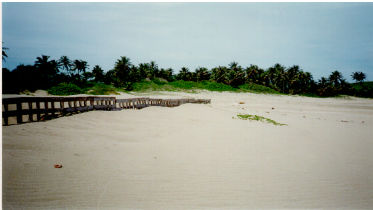
Photograph 5. Sand fence at Barceloneta, Puerto Rico, October, 1997. Note the fence has trapped sand so that the pallets are almost covered.
