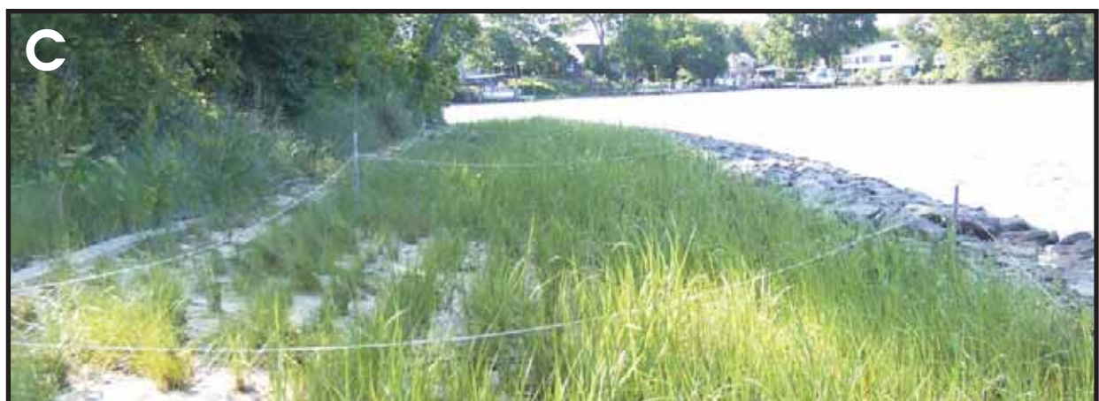
Figure 4-9. Hull Springs Farm shoreline A) before construction, B) after construction of the sill and placement of sand, and C) after planting.
