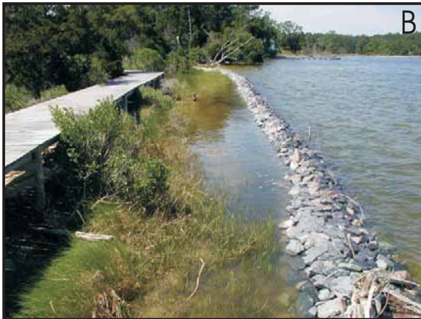
Figure 3-4. Photos showing marsh toe revetments A) before and B) after a project on Cranes Creek in Northumberland County and C) before and D) after a project on Mosquito Creek in Lancaster County, Virginia.
