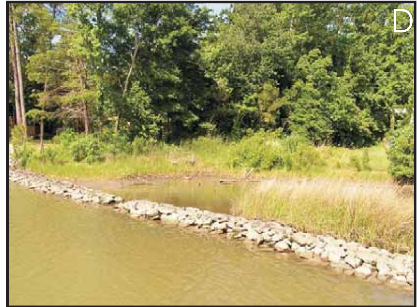
Figure 3-4. Photos showing marsh toe revetments A) before and B) after a project on Cranes Creek in Northumberland County and C) before and D) after a project on Mosquito Creek in Lancaster County, Virginia.
