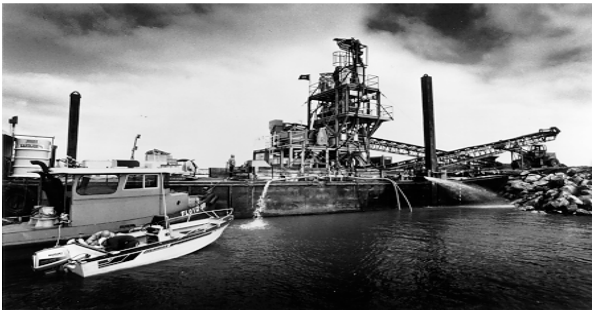
Bergmann Soil and Sediment Washing
