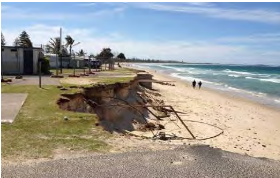
Figure 13 – Cable and Piping Infrastructure currents protruding from the erosion escarpment adjacent to the Holiday Park. Photo: M. Daley 8 November 2011.
