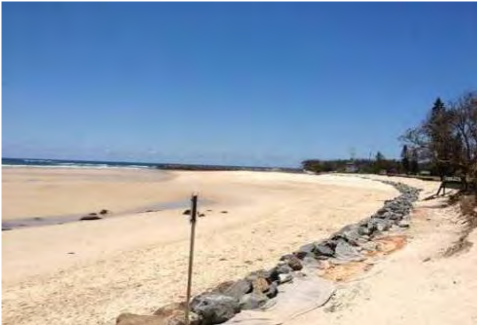
Figure 6 - Terminal rock revetment between Cudgen Headland SLSC and the Cudgen Creek training wall (present in the background). The photo shows the current sand pulse that has recently moved into the embayment and now resides at the southern end of the compartment in front of the wall. Photo M. Daley 8 November 2011.
