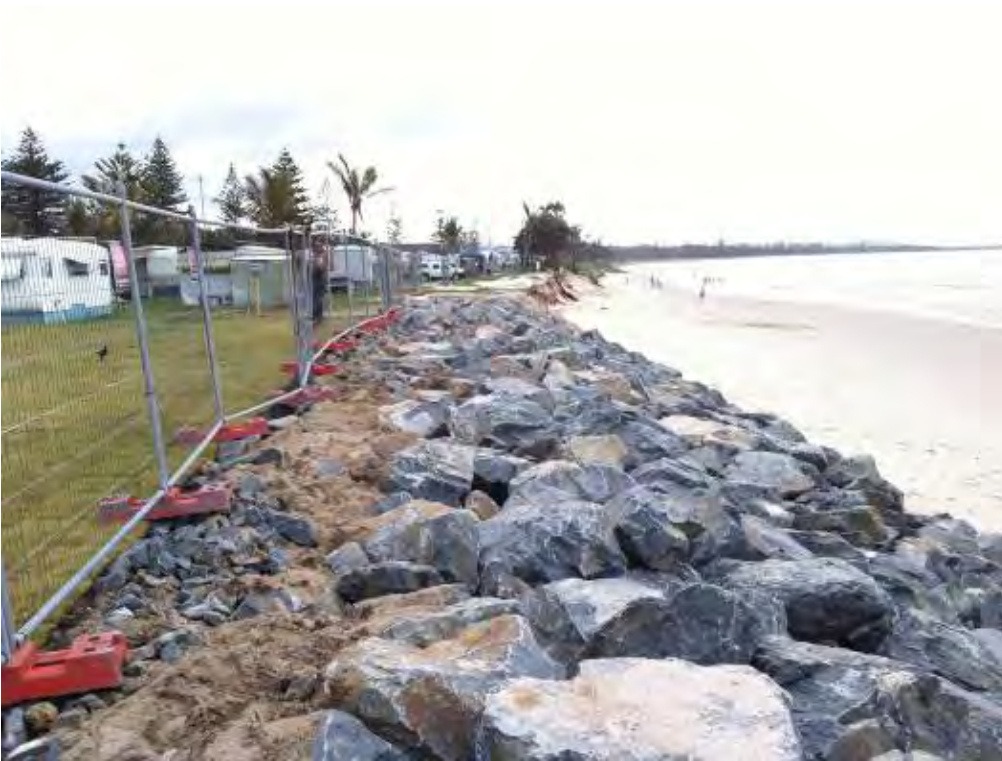
Figure 15 – Recent (December 2011) rock revetment works installed to protect the amenities block and sewer pumping station of the Kingscliff Holiday Park. Photo: B. Fitzgibbon 14 December 2011.
