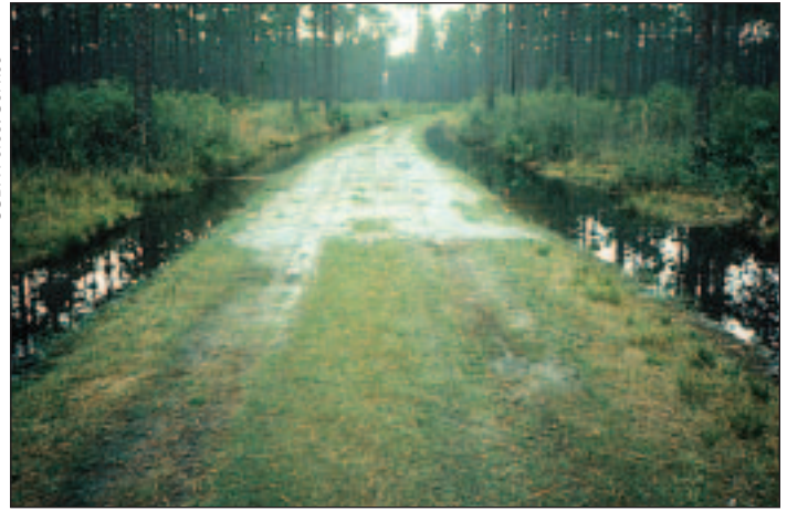
▲ Removal of the geotextile and expanded metal leave the road surface relatively undisturbed.
