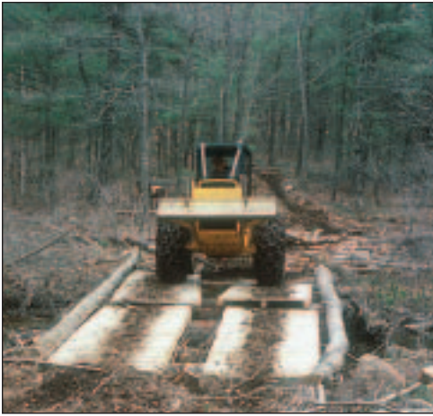
▲ Corduroy approaches help control erosion and keep mud off the logs and out of the stream.
