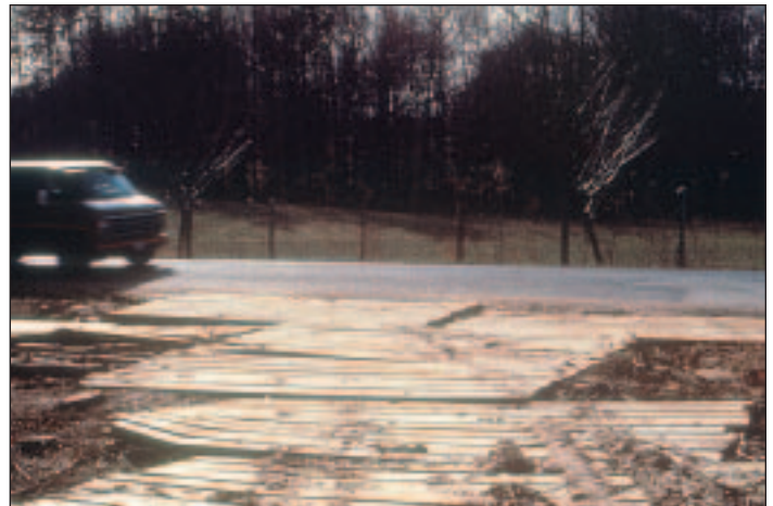
▲ Wooden mats can be used to provide mud-free highway approaches.
