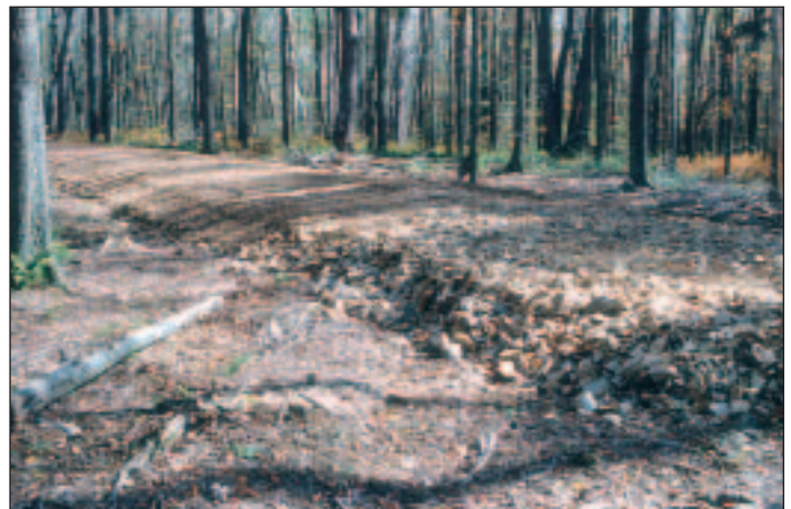
▲ Gravel surface may be used directly over chunkwood fill for a lightweight road where a porous section is less important.
