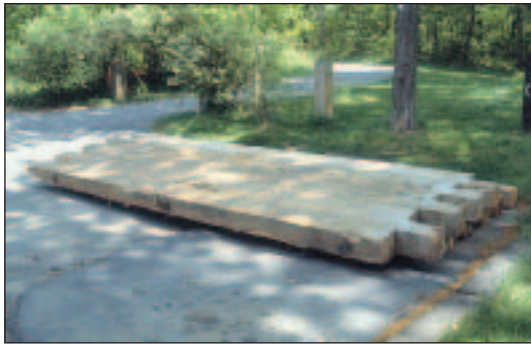
▲ The staggered-end design of this low-cost portable skidder bridge, built by John Conkey Logging Co., helps to keep it in position in use.
