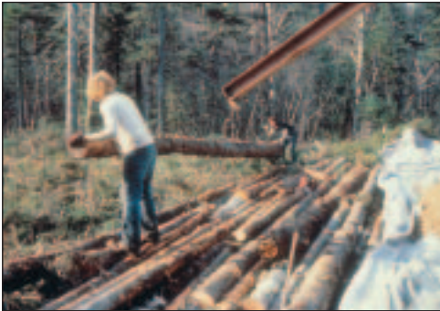
▲ A corduroy of parallel laying logs is placed on top of the geotextile.
