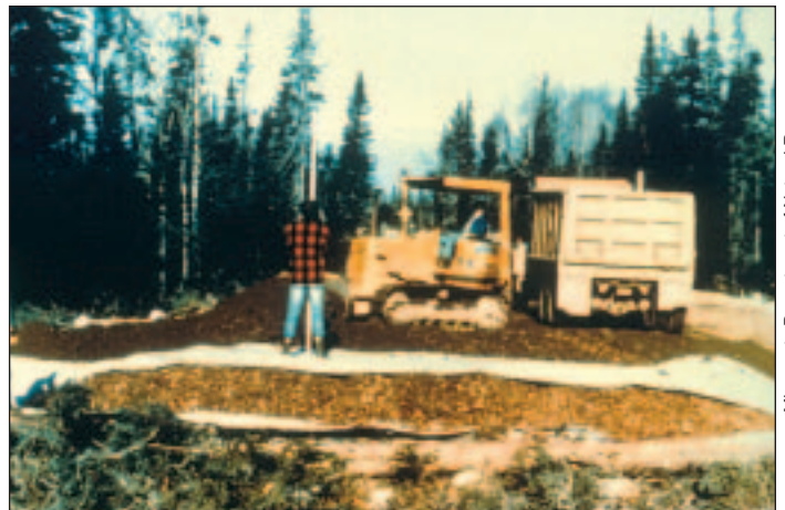
▲ Another layer of geotextile is placed on top of the chunkwood to prevent contmination and sealing of the porous layer. The gravel running surface is placed on top of the geotextile fabric.
